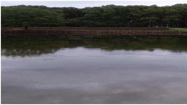
Fig. 3. Embankment behind the mangrove
