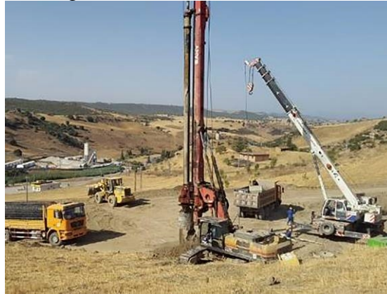
Fig. 7 Construction of green pile foundation
