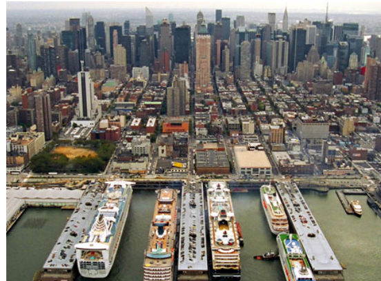
Fig.10 Aerial View of Manhattan Cruise Terminal's Pier 88-91
