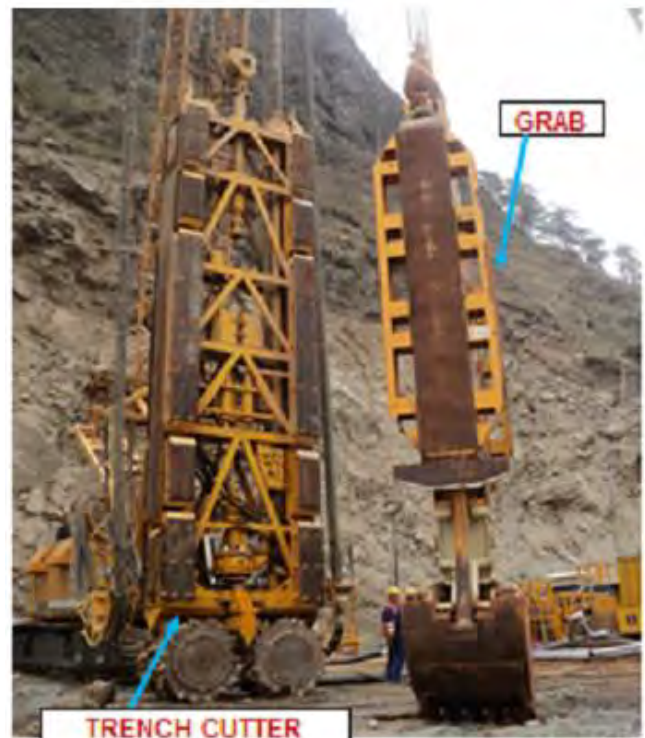
Fig. 3. A view of hydraulic trench cutter and grab
