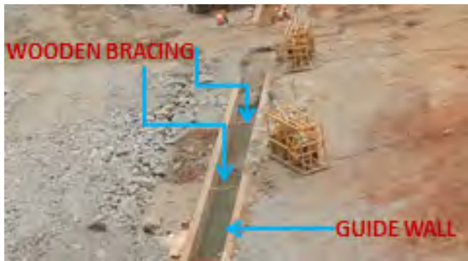
Fig.6. A view of guide wall with wooden bracings
