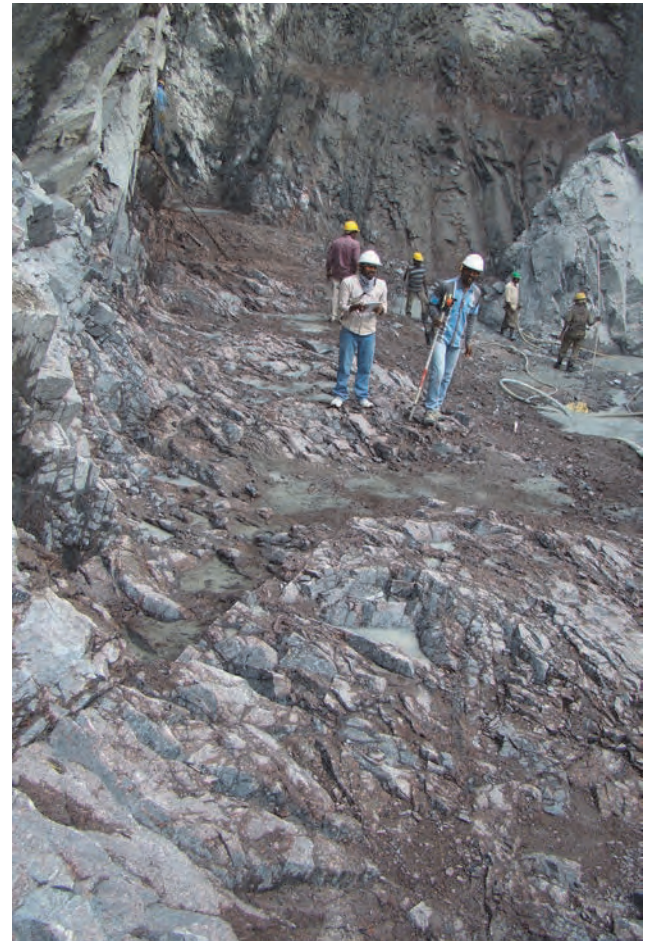
Fig. 4. Pink granite mapped at the foundation of pump house
