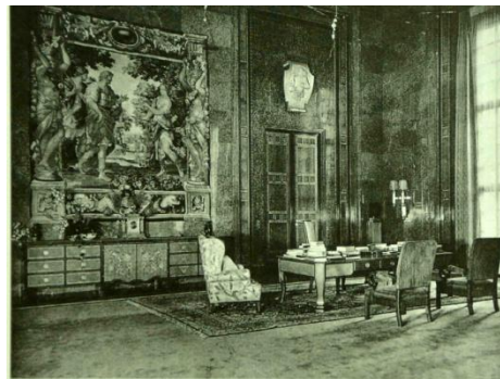
Fig. 19. Hitler’s Office, Premier House of the New Empire 1939
