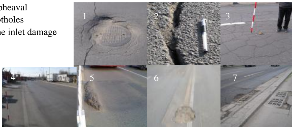
Fig.3 The main asphalt pavement diseases
