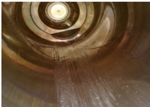
Figure 1. Scratch on the surface of hydraulic cylinder bore
