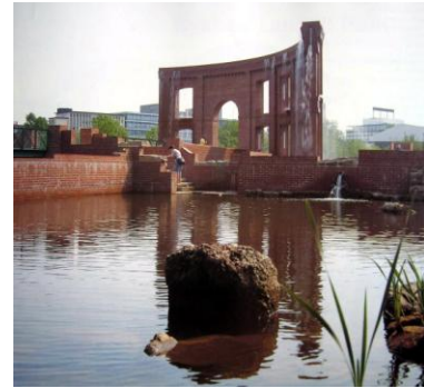
Figure1. The water tower where surface water drainage from the site is collected and cascaded in order to oxygenate it.[4]
