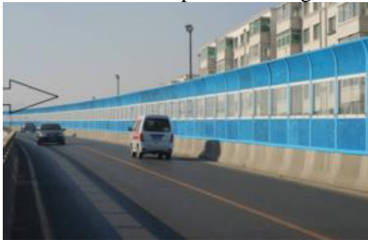
Fig.15 Aluminium foam sound barrier in shenyang
