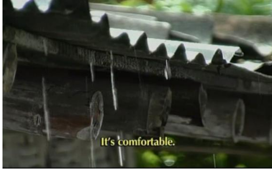
Fig. 6. Raindrops on the roof
