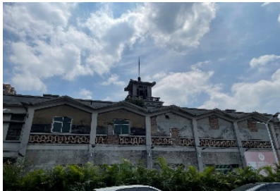
Fig. 2. Real view of the back of the building
