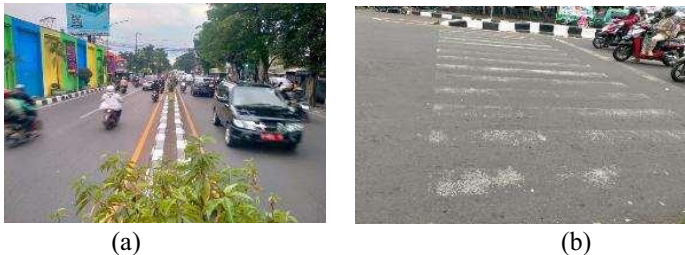
Fig 3 (a) Median on the road at Phh Mustofa Street. (b) Zebra crossing on Phh Mustofa street.
