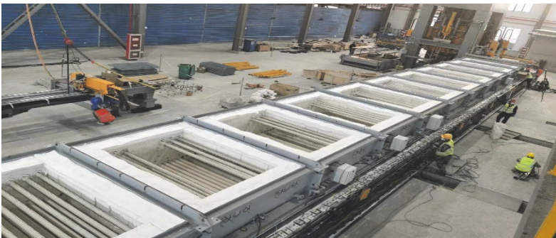
Fig. 5. Heating furnace insulation and components installation process
