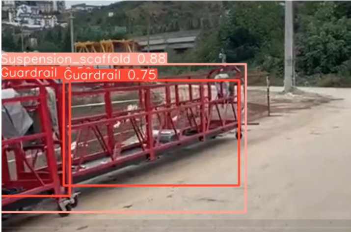
Fig. 4. Suspension scaffold and Guardrail detections after model training
