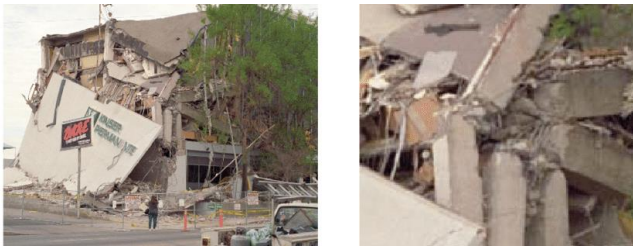
Figure 1. Building Collapsed due to connections failures [4]
