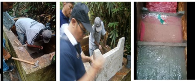
Figure 5. Installation of filters and filter media
