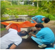
Figure 13. Installed the batteries
