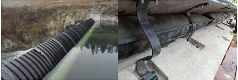
Figure 1. Pneumatic crest gate front and rear view
