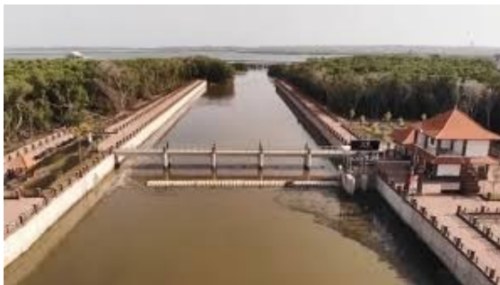
Figure 3. Mati river movable dam with pneumatic crest gate system
