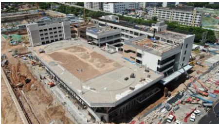
a) before covering the sports field with soil and grass
