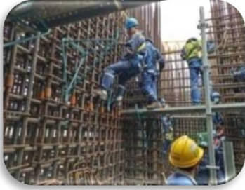
Fig. 11. Manual binding of steel bars
