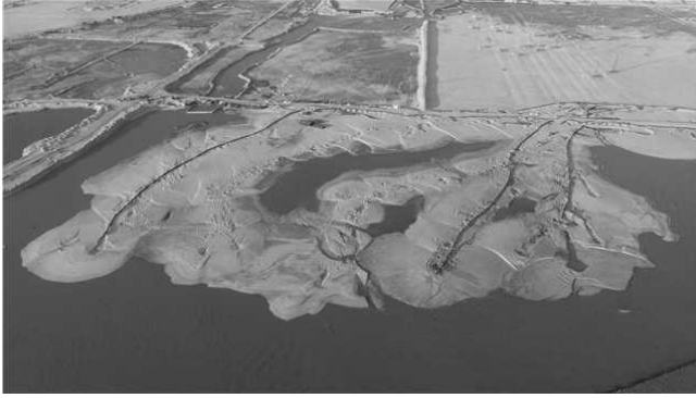
Fig. 1. Xiamen New Airport Reclamation Project
