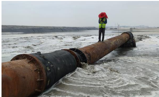
Fig. 7. Connecting rubber pipe at the male port and connecting steel pipe at the female port
