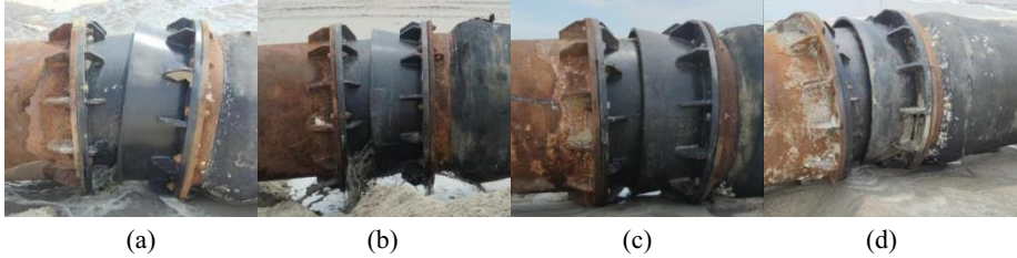
Fig. 8. Connecting rubber pipe at the female port and connecting steel pipe at the male port
