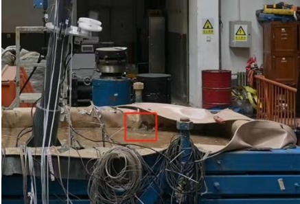
(a) Water bubbling up from sandblasting on the soil surface
