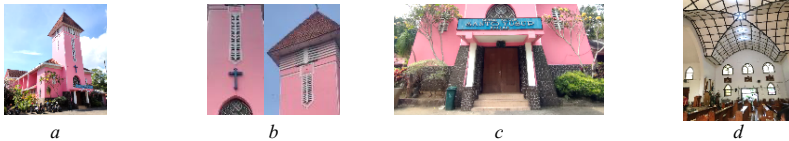
Figure 3 St. Yusup Blitar Church showing (a) the facade of the building, (b) roof and ornamentation, (c) doors, walls and columns, (d) ribbed vault
