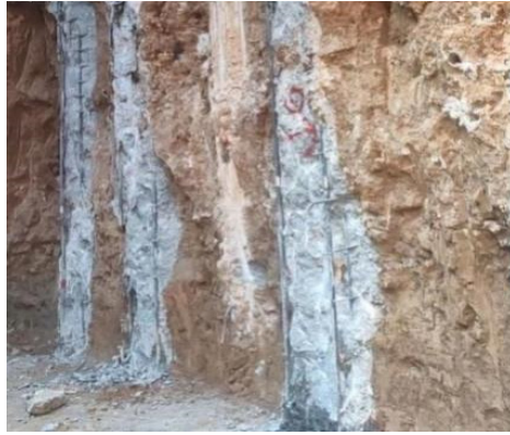
Fig. 4. On-site chiseling of pile foundation protective layer
