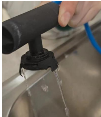
Fig. 4. Condition of fire water flow
