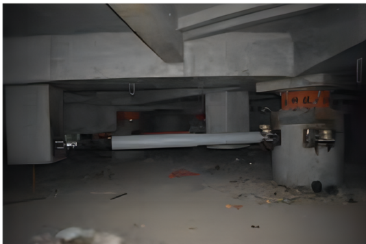
Fig. 4. Installation of viscous damper in isolation layer [37]
