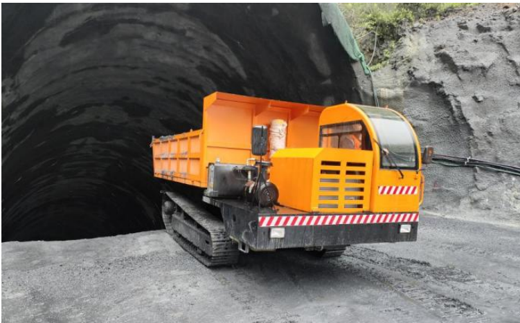
Fig. 10. Operation of the Tracked Dump Truck for Slag Discharge.
