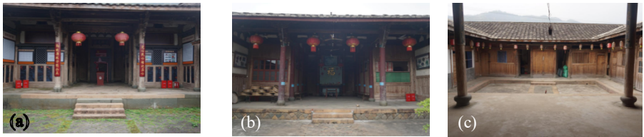
Fig. 9. The repaired historic building
