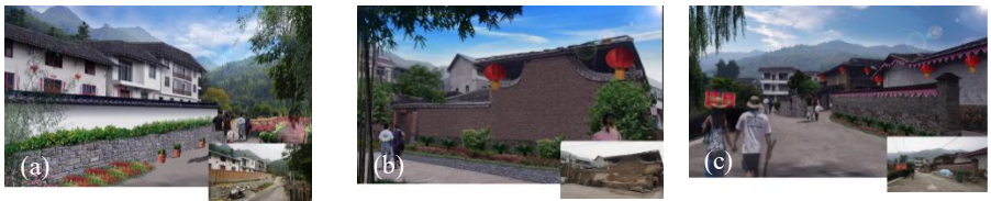
Fig. 10. The renovated street and alley
