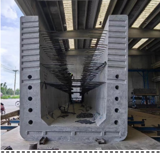
Fig. 5. Prefabricated U-shell segments
