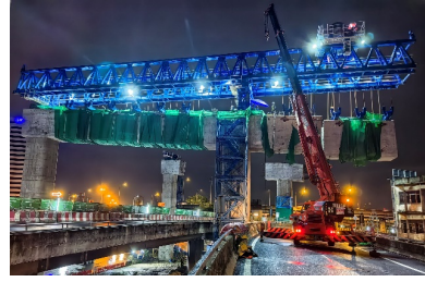
Fig. 6. Segment block alignment
