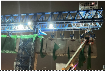
Fig. 7. Tensioning temporary prestressing on the outside of the U-shell
