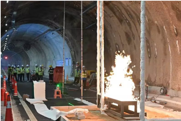
Fig. 5. Small scale fire test of foot tunnel
