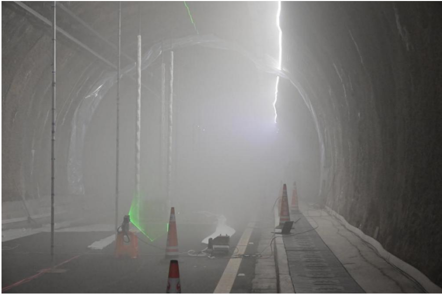
(a) Before the start of the "one-key linkage" control plan for the tunnel electromechanical equipment (the flue gas is not discharged from the tunnel)
