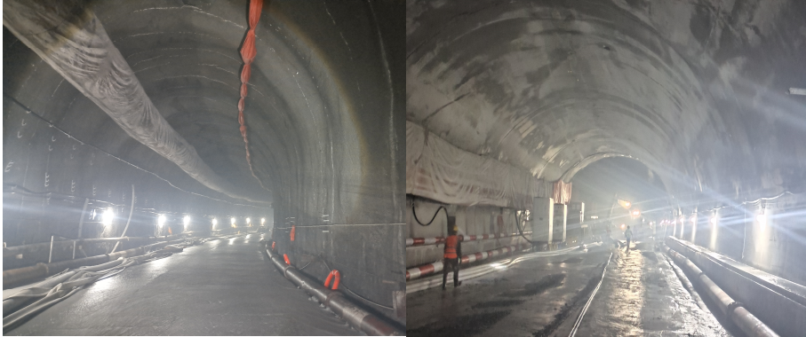
a) Completion of Slope Draining
