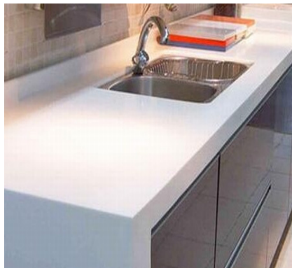
Fig. 2. Seamless splicing of synthetic stone on kitchen countertops. (Source of the picture: https://zhishi.fang.com )
