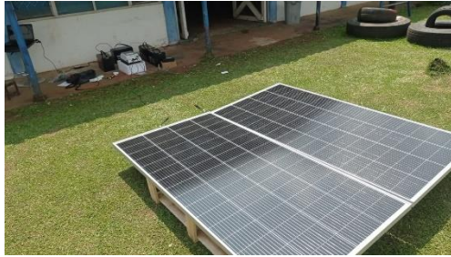
Figure 7. Solar panel testing
