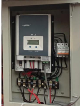
Figure 2. Installation of MPPT and electrical components
