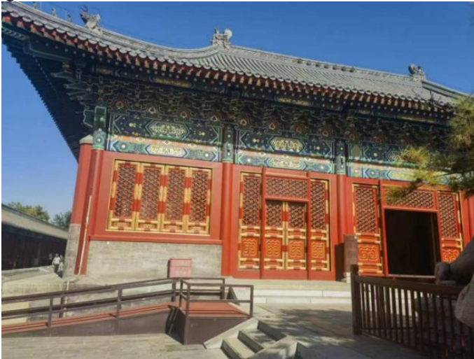
Fig. 4. Roof of the main hall
