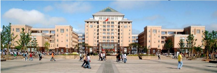
Fig. 1. Comprehensive Teaching Building
