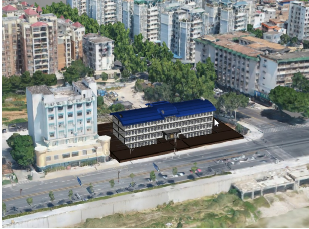
Fig. 3. Result of the exterior of the Office Building and oblique photography data
