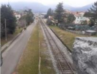
Fig. 1: The cross-border area of San Gabriele right on the border, standing on the tunnel of the railway
