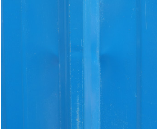
Fig. 9. Damage consequence of 100 g explosive plate
