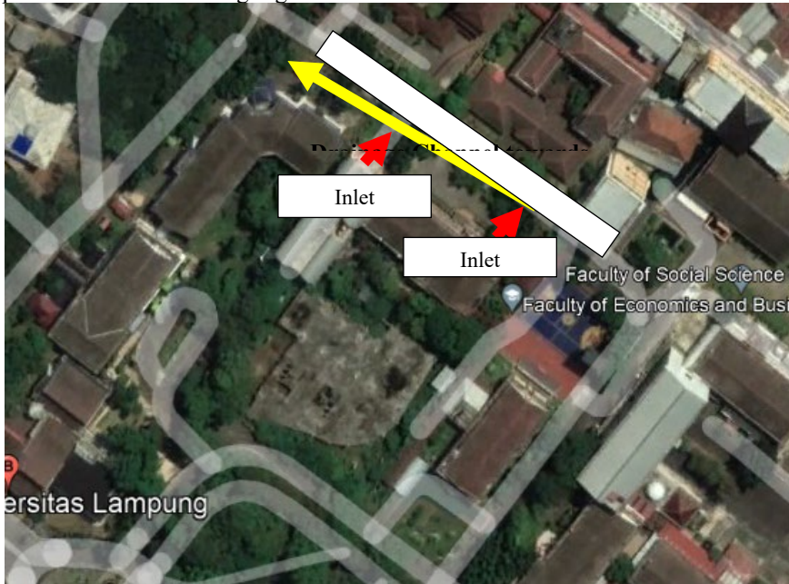
Fig. 4. Water flow in drainage channels.
