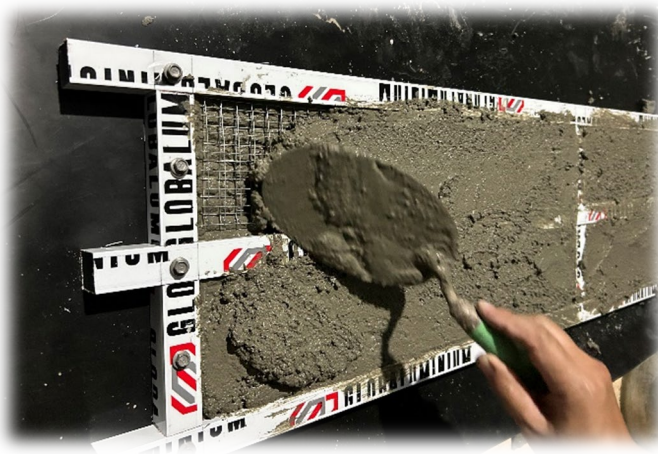
Fig. 4. Formwork and reinforcement.
