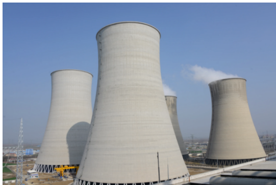
Fig. 8. Cooling tower of a certain power plant.
