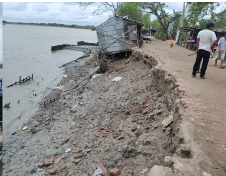
Fig. 6. River Bank Erosion
