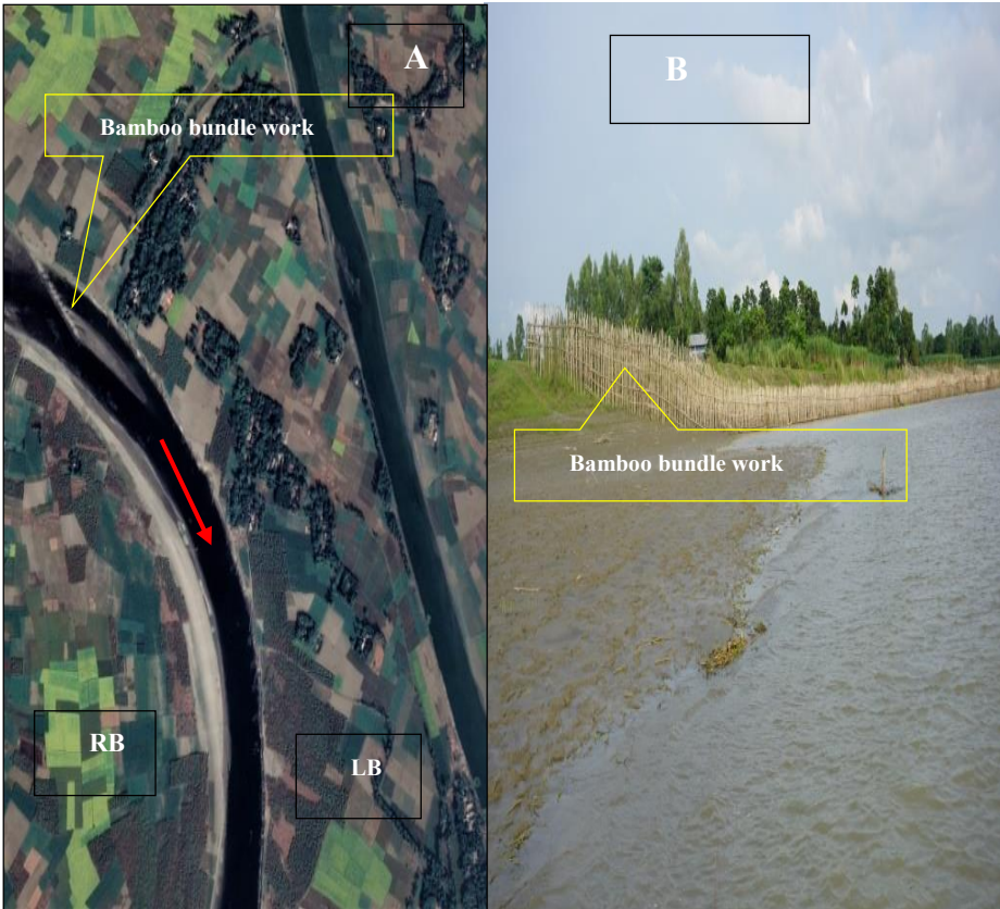
Fig. 8. Picture (A) planform view of bamboo bundle work Google image 2018 work and picture (B) field image of bamboo bundle work along left bank of Old Brahmaputra River.
