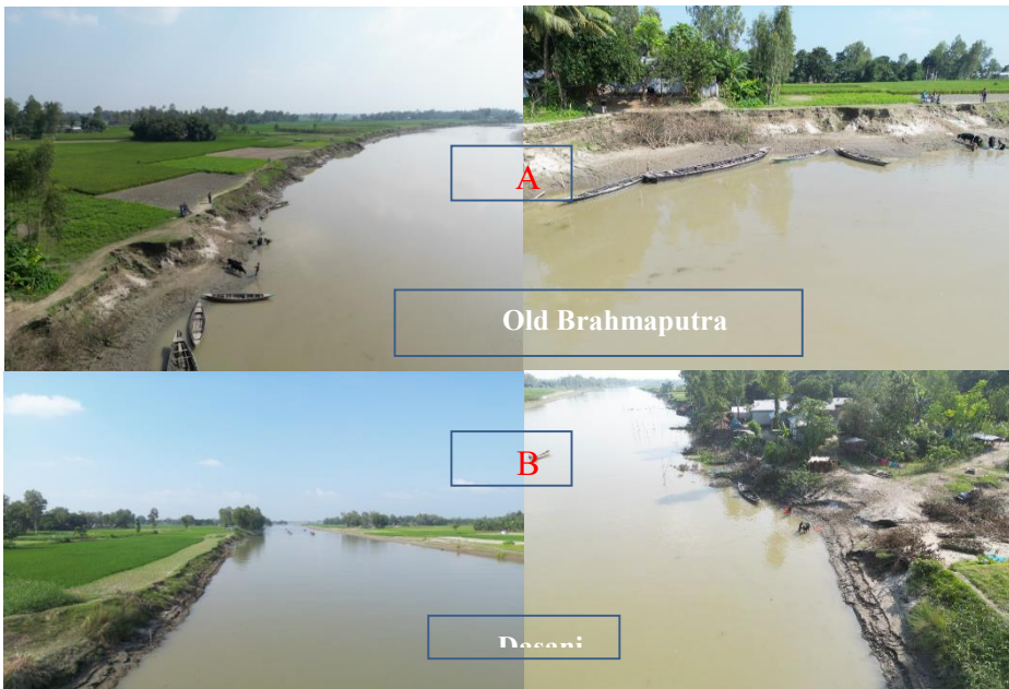
Fig. 10. Pictures of Old Brahmaputra (A) and Dasani (B) River bank erosion near at Bakshiganj upazila in Jamalpur district (20/10/2023).
