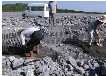
d. Dig the reinforcement
