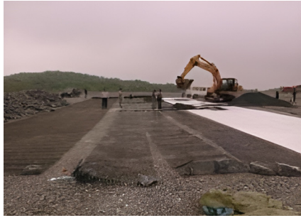
a. Lay reinforcement and protective layer
