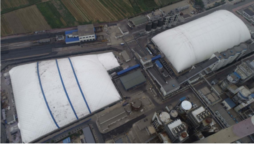
Fig. 1. Real picture of an air-supported structure in a power plant
