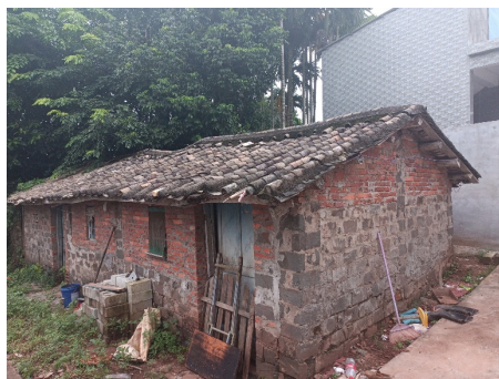
Fig. 13. brick-stone mixed structure in Hainan Province
