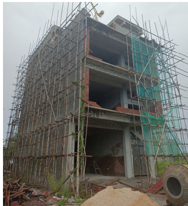
Fig. 19. A framework structure under construction in Hainan Province
