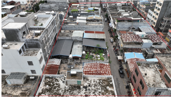
Fig. 6. Aerial photo of brick-concrete structures in Lincheng town, Lingao County
