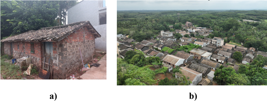
Fig. 5. Brick-stone mixed structure and the aerial photography of brick-wood structures in Shimengao Village
