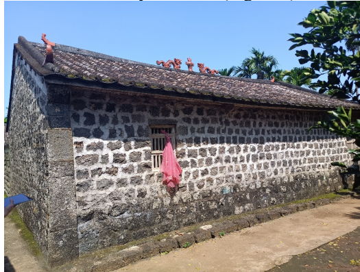
Fig. 8. Stone-wood structure of Hainan Province
