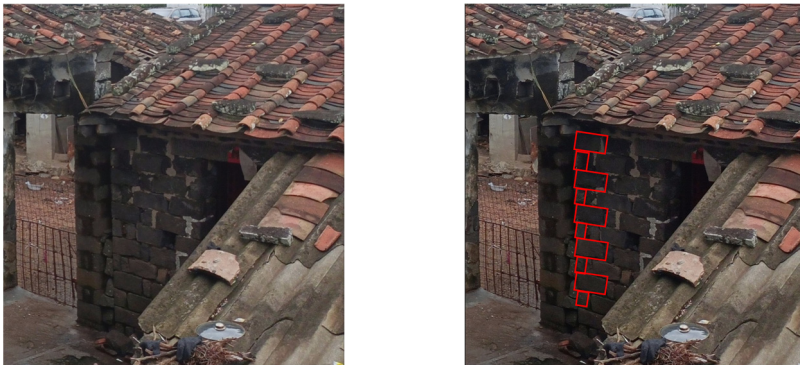
Fig. 11. Schematic diagram of stone-wood structure interlocking masonry in Hainan Province
