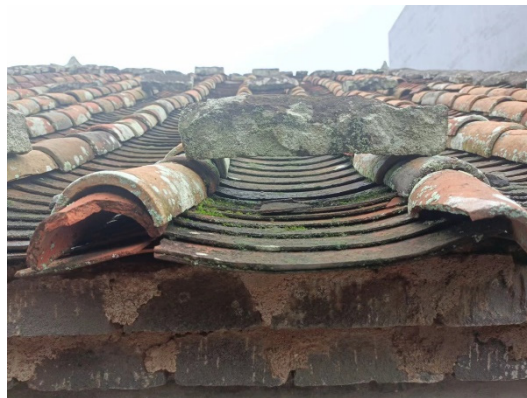
Fig. 9. Detailed drawing of the Chinese style tile on the top of the stone-wood structure in Hainan Province
