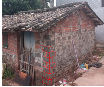
Fig. 15. interlocking masonry of the brick-stone mixed structure
