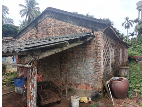
Fig. 14. Brick-wood structure in Hainan Province (cavity wall)
