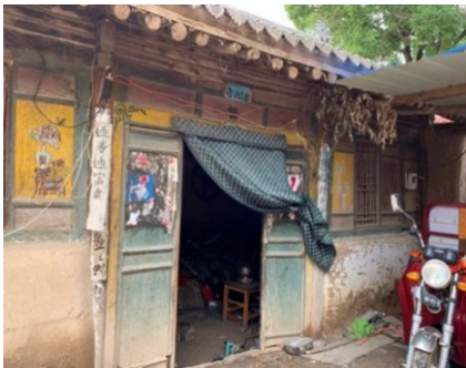
(c) Inverted utility room
