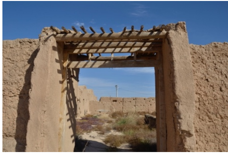
Fig. 12. Photo of the entrance gate of the courtyard .Source: Self-taken
