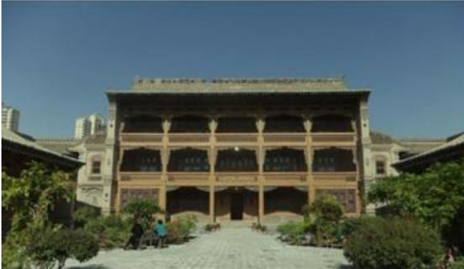
Fig. 1. Actual view of wooden building cover structure
