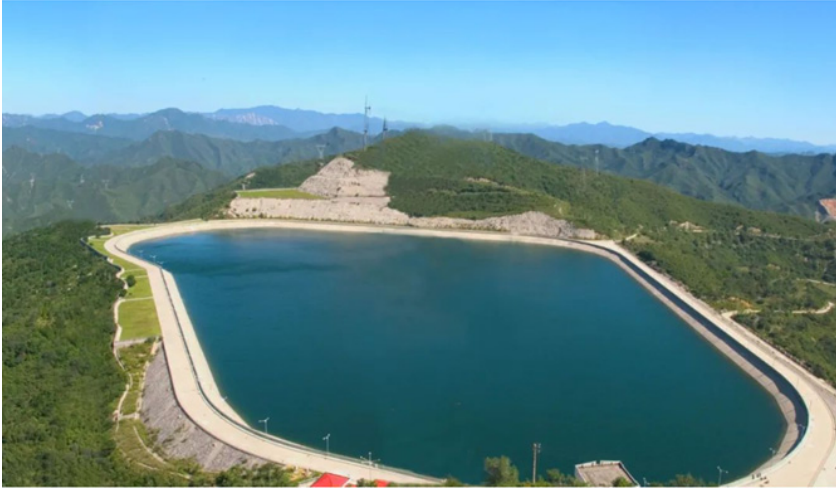
Fig. 3. Upper reservoir of a pumped storage power station (This image comes from the Internet)
