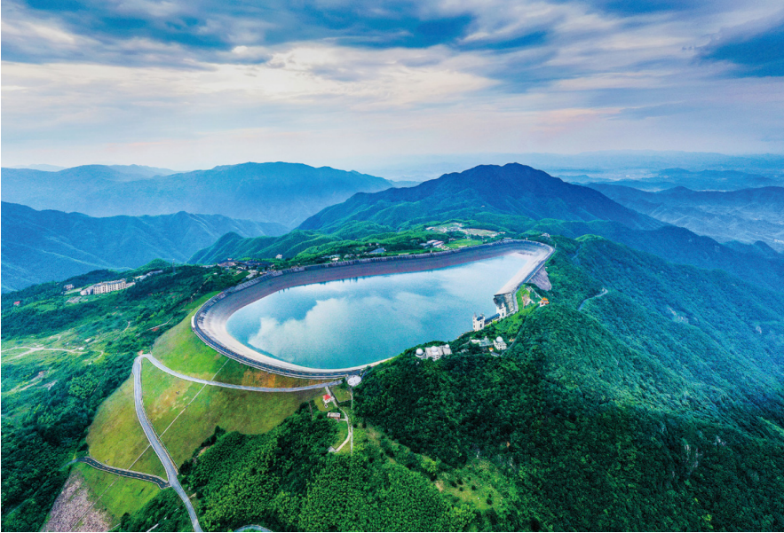
Fig. 5. Upper reservoir of a pumped storage power station (This image comes from the Internet)
